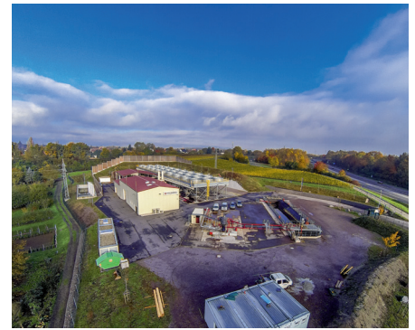
Fig. 6 Geothermal power plant Insheim (Source: Pfalzwerke geofuture GmbH)
